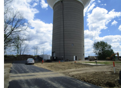
Final site work is underway and asphalt driveway installed.
