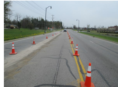
Crews grind off existing stripping to make way for a new turn lane.
